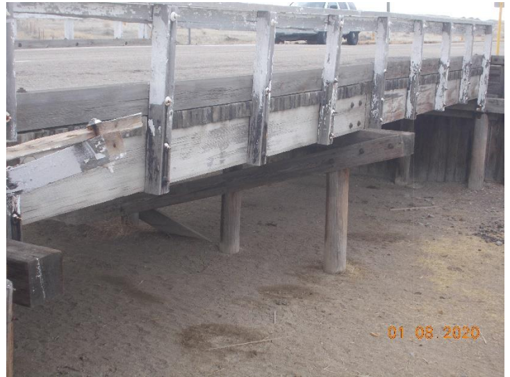
Side view of bridge M-21-J.
