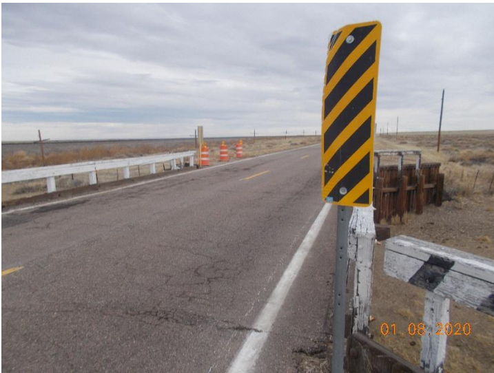
View of bridge M-21-J looking northeast.
